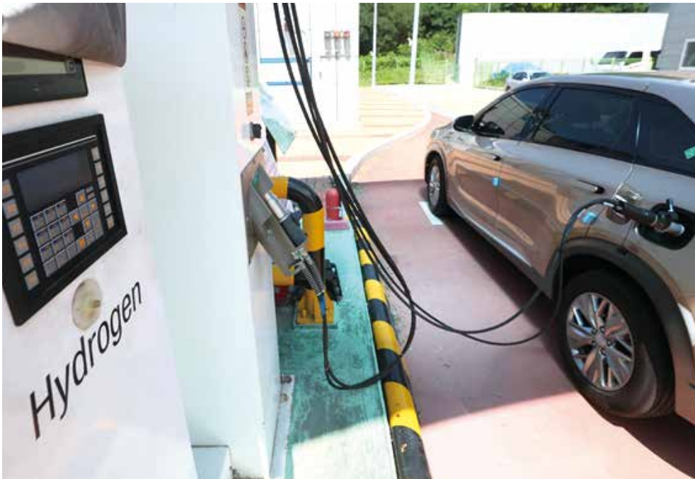
Hydrogen car charging station in Mapo-gu, Seoul 34
